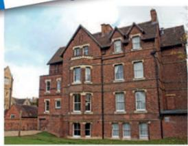
Complete refurbishment of four-storey villas on Bradmore Road to provide updated student accommodation. A fast-track project with prefabricated en-suite pod bathrooms, soundproofing and DDA improvements
